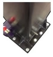
6. Ensure top plates are installed on posts and bolts are tightened.
