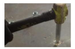
5. Move posts back into position over holes and insert bolts to secure posts to floor.
