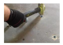
4. Expand inserts with driver to secure in hole
